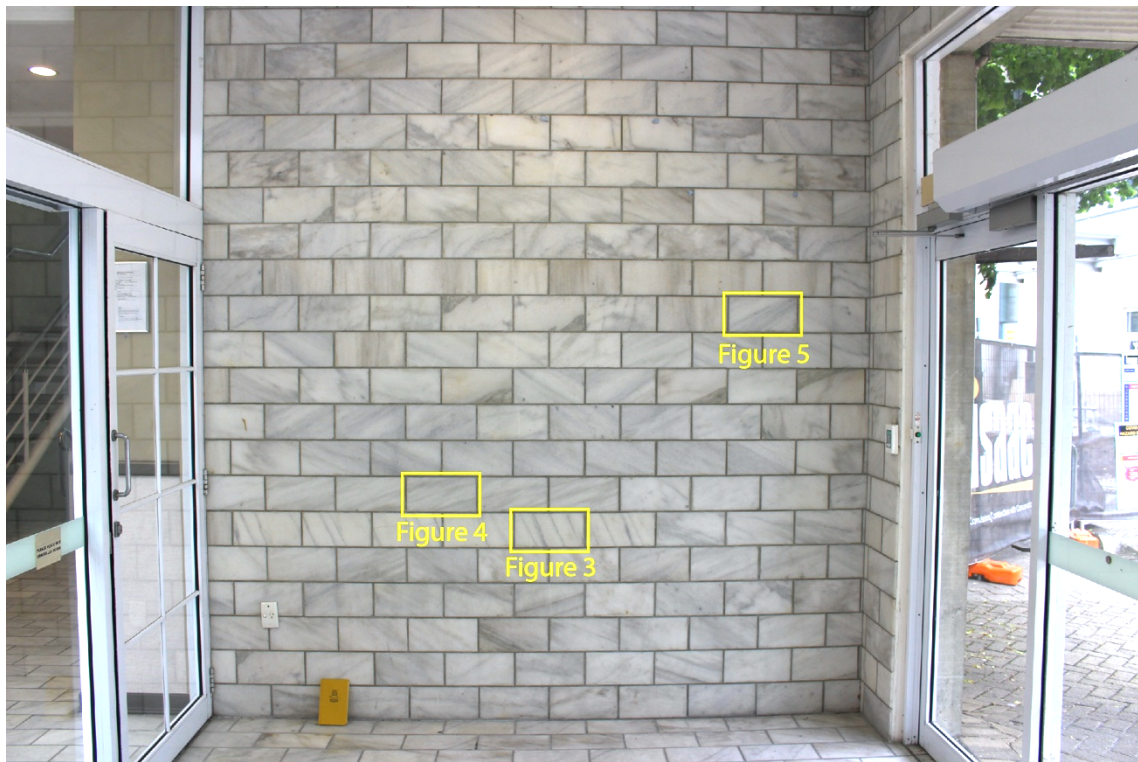
Figure 2: Marble wall tiles inside main entrance (west) to the Castle Lecture Theatres.
