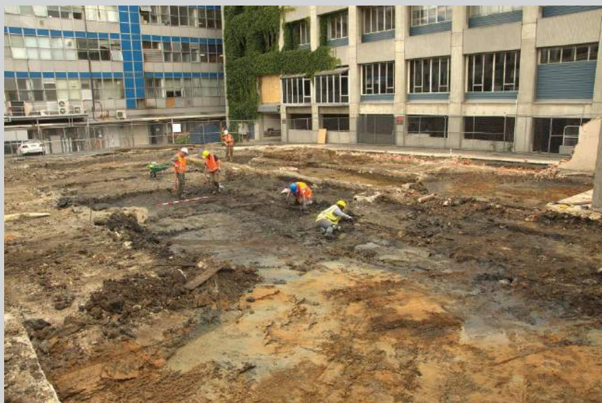
Archaeology staff examine the site of the former Barningham Building for relics of early Dunedin as part of the Dental School redevelopment.
