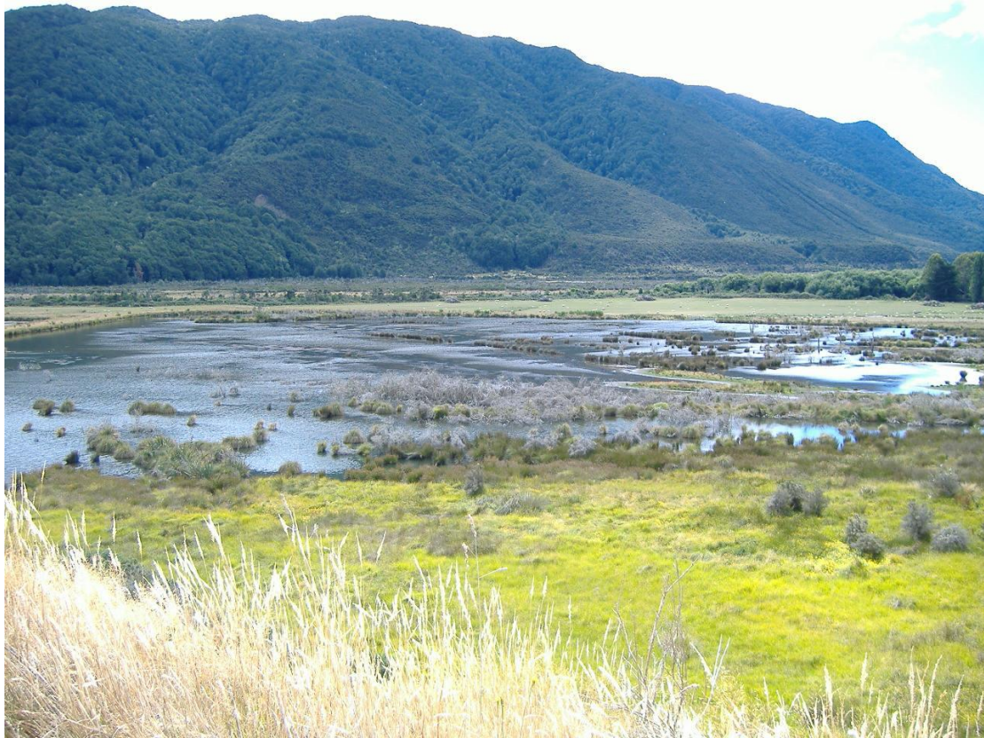
Figure 1. Photo of SS1 pond showing an example of pond being constructed with a dam (at far right).
