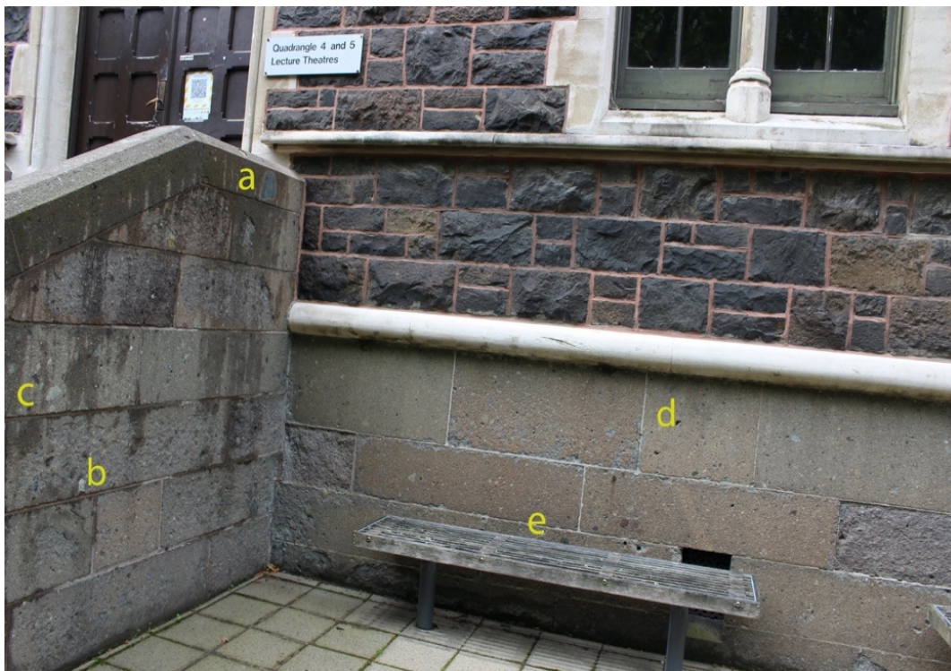
Figure 1: Front façade of the Geology Building showing Port Chalmers breccia that makes up the stairs and the lower part of the front wall (underneath the light colored Oamaru Limestone.). The letters refer to the individual clasts shown in Figure 3.
