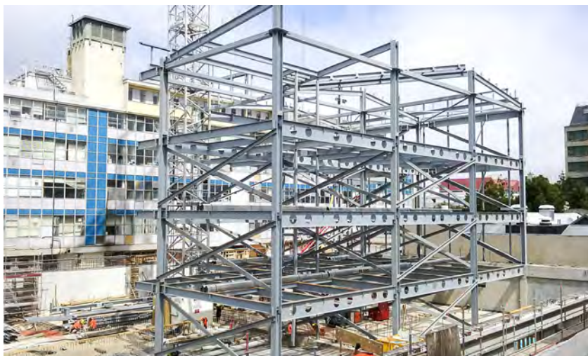
Clinical Services Building under construction, November 2017.
