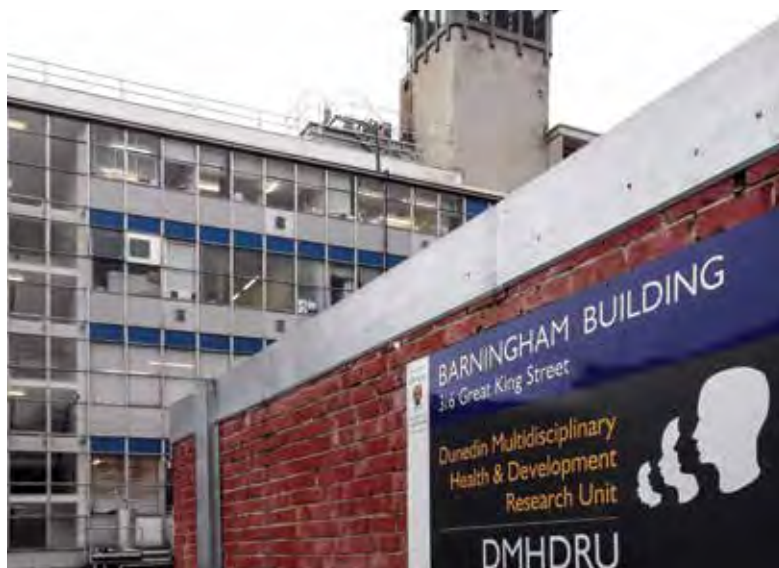
The Barningham building, former home of the Dunedin Multidisciplinary Health and Development Study, adjoining the west wing of the Walsh Building. Both were demolished in 2016 to make way for the new Clinical Services Building of the Faculty of Dentistry. As of late 2016 the Dunedin Study is based at Logan Park, while a new $2.6M facility is built for the Study in Anzac Avenue near the University's premises at Forsyth Barr Stadium.
