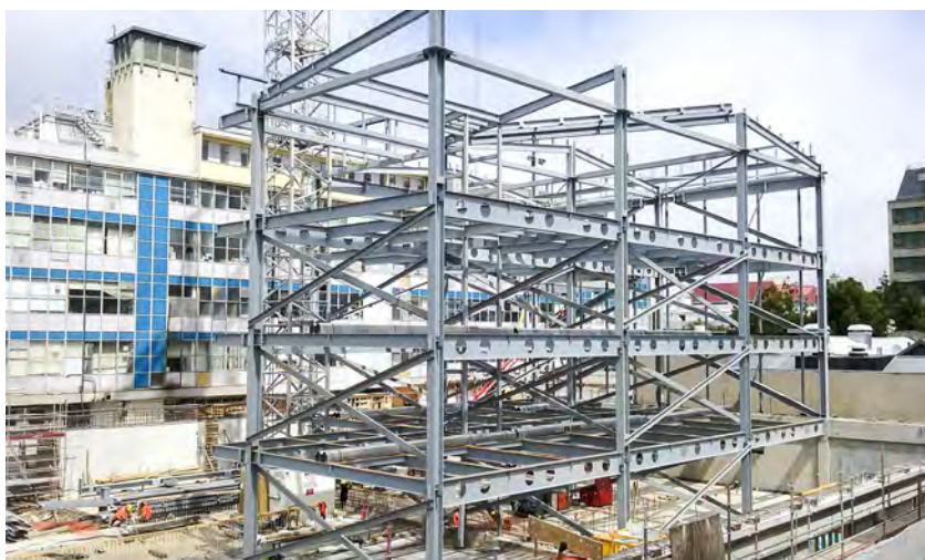
Clinical Services Building under construction, November 2017.
