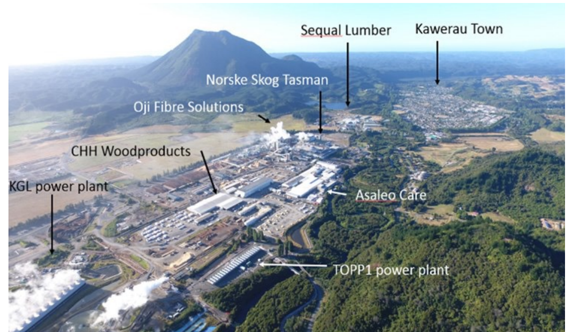
Figure 2: Kawerau Industrial Complex [2]
