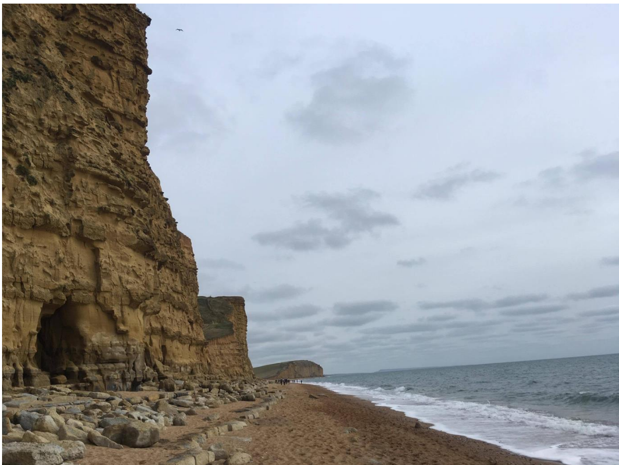
The Bridport Sand Formation observed at a cliff face at West Bay, Dorset.
