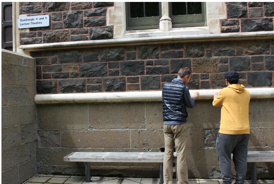
Figure 1: Oamaru Limestone is one of rock types used to build the Geology Department. The limestone is visible as light, cream-coloured rock.
