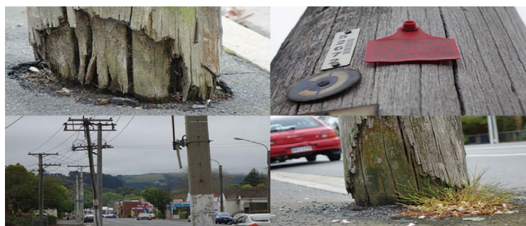
Rotting power poles in Otago.
