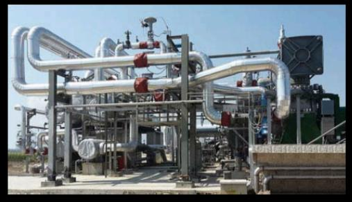
Possible to use organic Rankine cycle (ORC) to generate electricity at low temperature ~100°C
