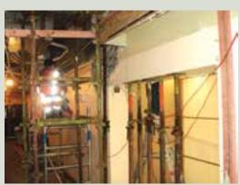
The damage and repairs to the University of Otago, Christchurch building. Walls were removed and opened up to check for unseen damage; epoxy resin pumped in to strengthen walls and floors; and stairwells rebuilt to stronger new standards.
