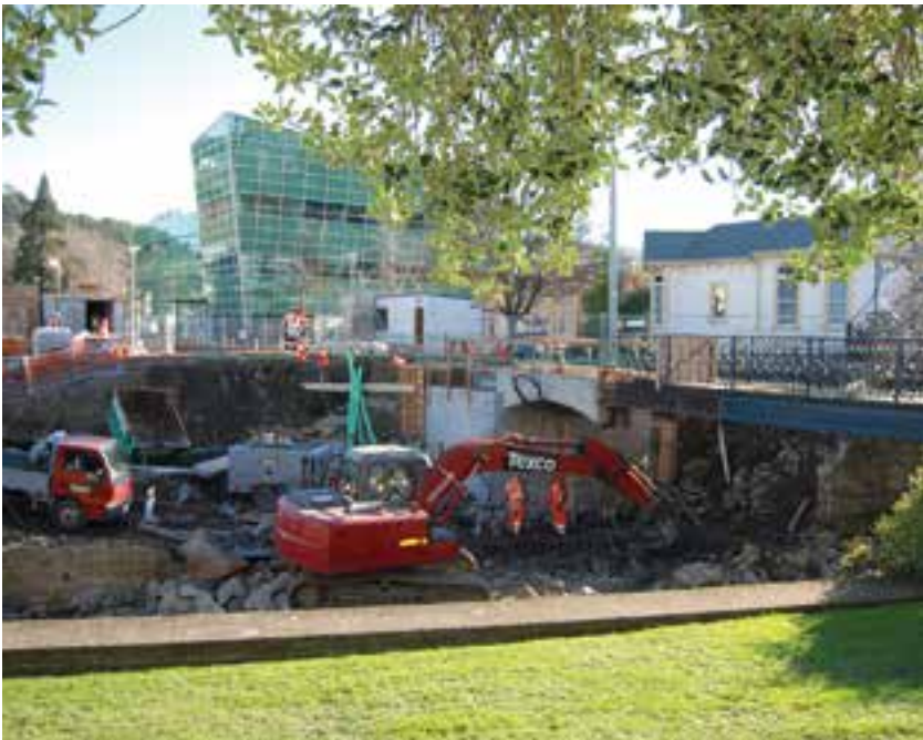
The St David footbridge was extended to allow a riverside path to pass beneath it.
