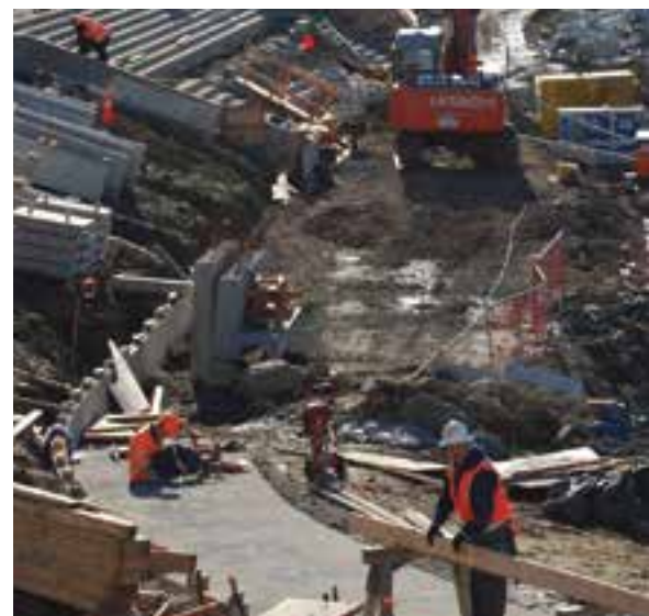
During: the western retaining wall has been demolished to make way for new terracing and steps down to the stream.
