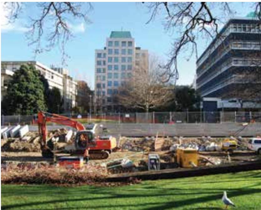
During: the western retaining wall has been demolished to make way for new terracing and steps down to the stream.
