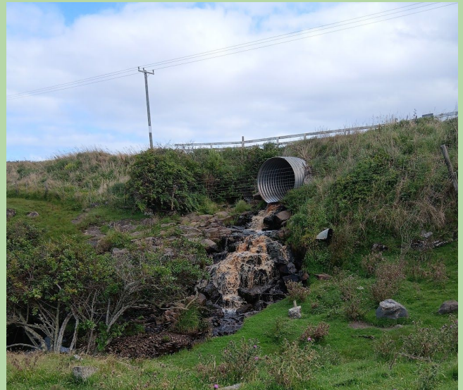
Man-made migration barrier (culvert) at Gillespie Stream.
