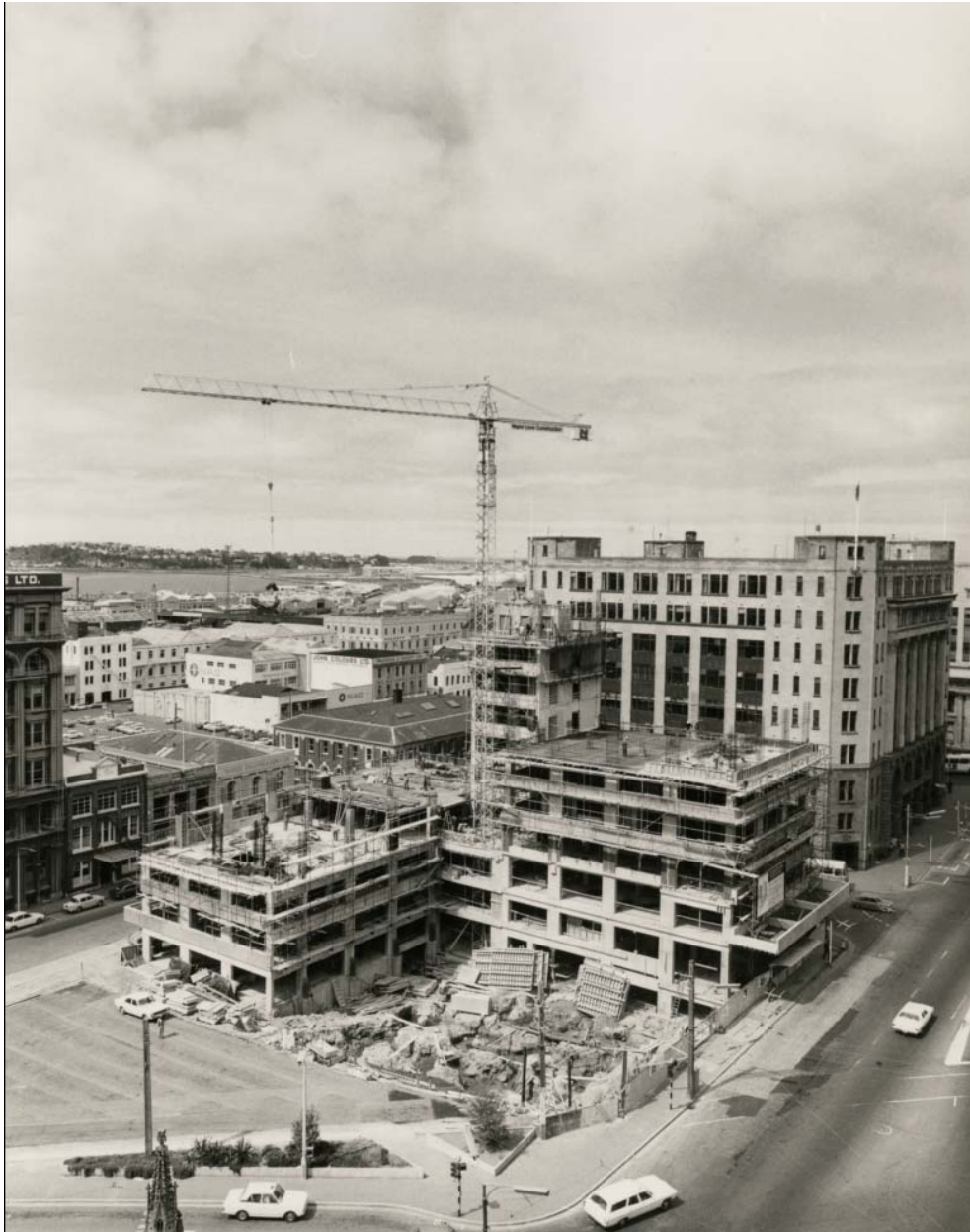
No. 827. John Wickliffe House, photographs of building during construction, 261-271 Princes Street, Dunedin, I.G. Dunn architect, Dalziel Architects records, 1974-1976, MS-2931/090, Archives & Manuscripts Collection, s14-543b.
