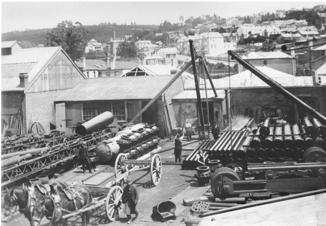
Cossens & Black's yard, Dunedin, c.1900, with new iron pipes for Central Otago gold sluicing prominent [c/n E953/42A]
