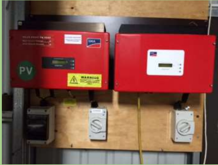
Car Battery to grid inverter
